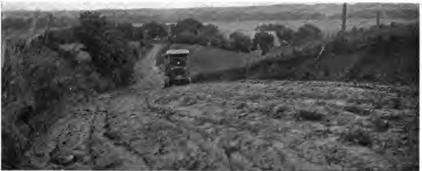
With this hill too much work has been put into widening the cut and not enough into reducing the grade. The grade is so stiff that local traffic cuts back and forth from side to side to relieve the horses, as shown by the various and curving ruts.
